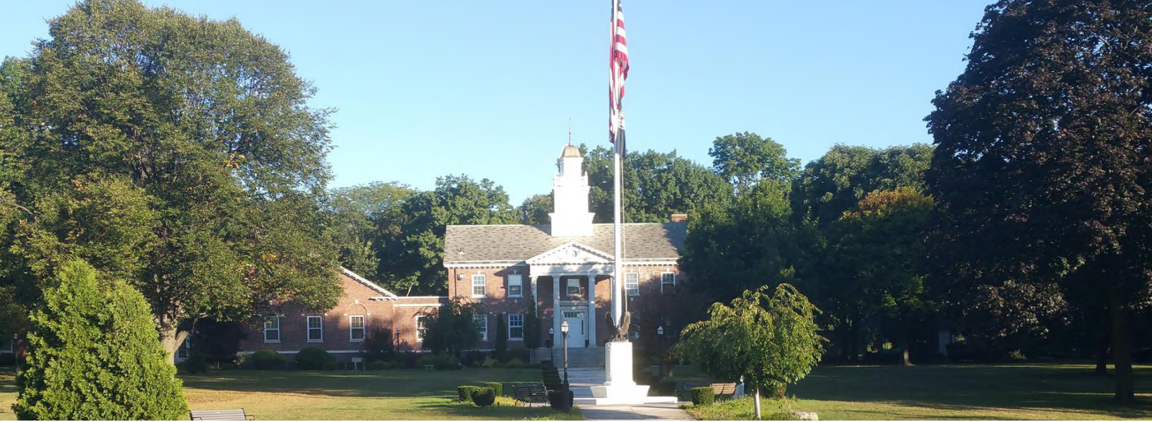
Photo: Municipal Building
